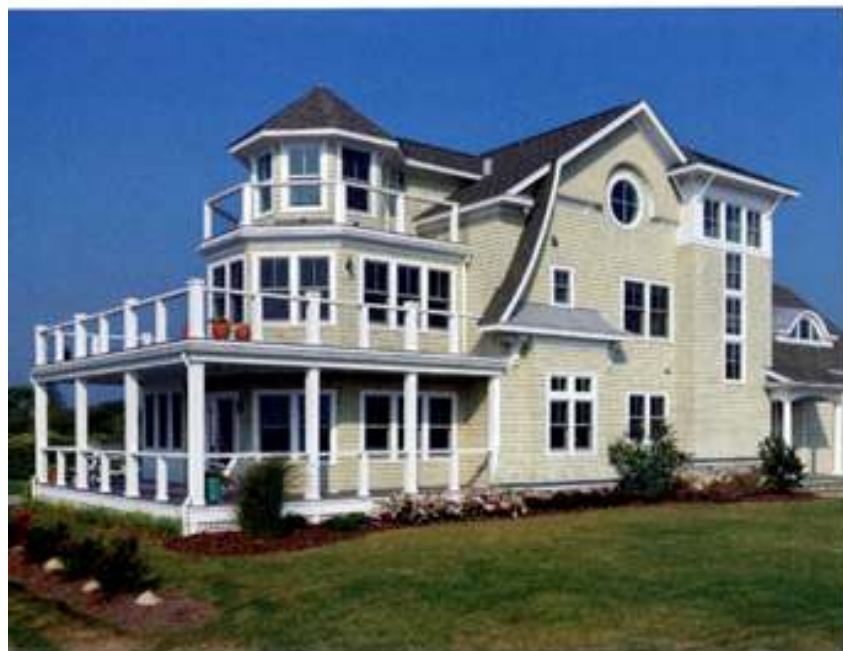
TOP: Red cedar shingles were bleached and dipped in stain at the factory to withstand the harsh elements. "They'll never rot in Ray's lifetime," Larson says. OPPOSITE TOP: Stones for the fireplace surround were gathered from the beach nearby, mimicking the look of the old cottage's fireplace. OPPOSITE BOTTOM: The open kitchen and generous pantry make cooking for family gatherings easy and fun.
